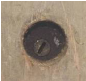
Lock Cylinder Removed
