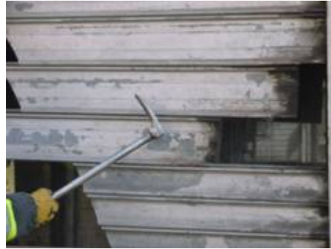
Drive Pike of Halligan into Slat to Remove
