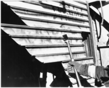
Drive Pike of Halligan into Slat to Remove
