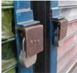
Welded Lock Cover
